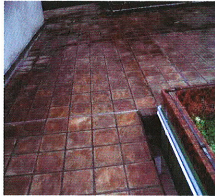
Photo A3-1 Concrete tiles, Roof of coffin crematorium building
