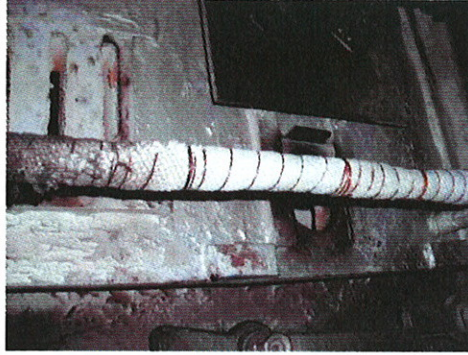
Photo A3-57 Insulation cloth/rope, Handle bar in Skeletal Room.
