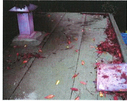
Photo A3-58 Bitumen Roof Felt, Roof of skeletal cremator building
